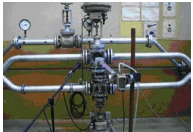
Fig. 8e: Real-time test rig at SAMSON AG
