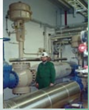
Team work is highly important to Jørn Møller (fifth from the right), head of SAMSON Denmark: The 2004 sales meeting was held on a sailing ship. · Over 30,000 versions can be assembled in Birkerød at short notice. · Jesper Petersen, a member of staff, starts up a control valve in a thermal power plant.
