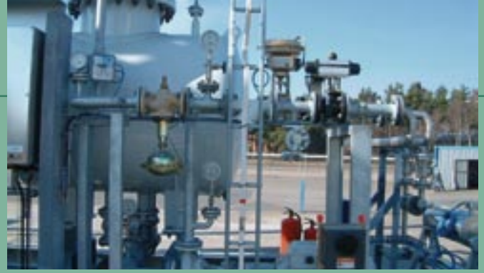
Cool Sorption uses SAMSON's self-operated regulators, control valves, positioners, and butterfly valves in its compact vapor recovery units.
